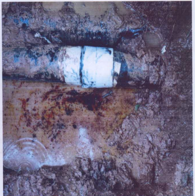
Fig E: Incident facility shortly after repair
